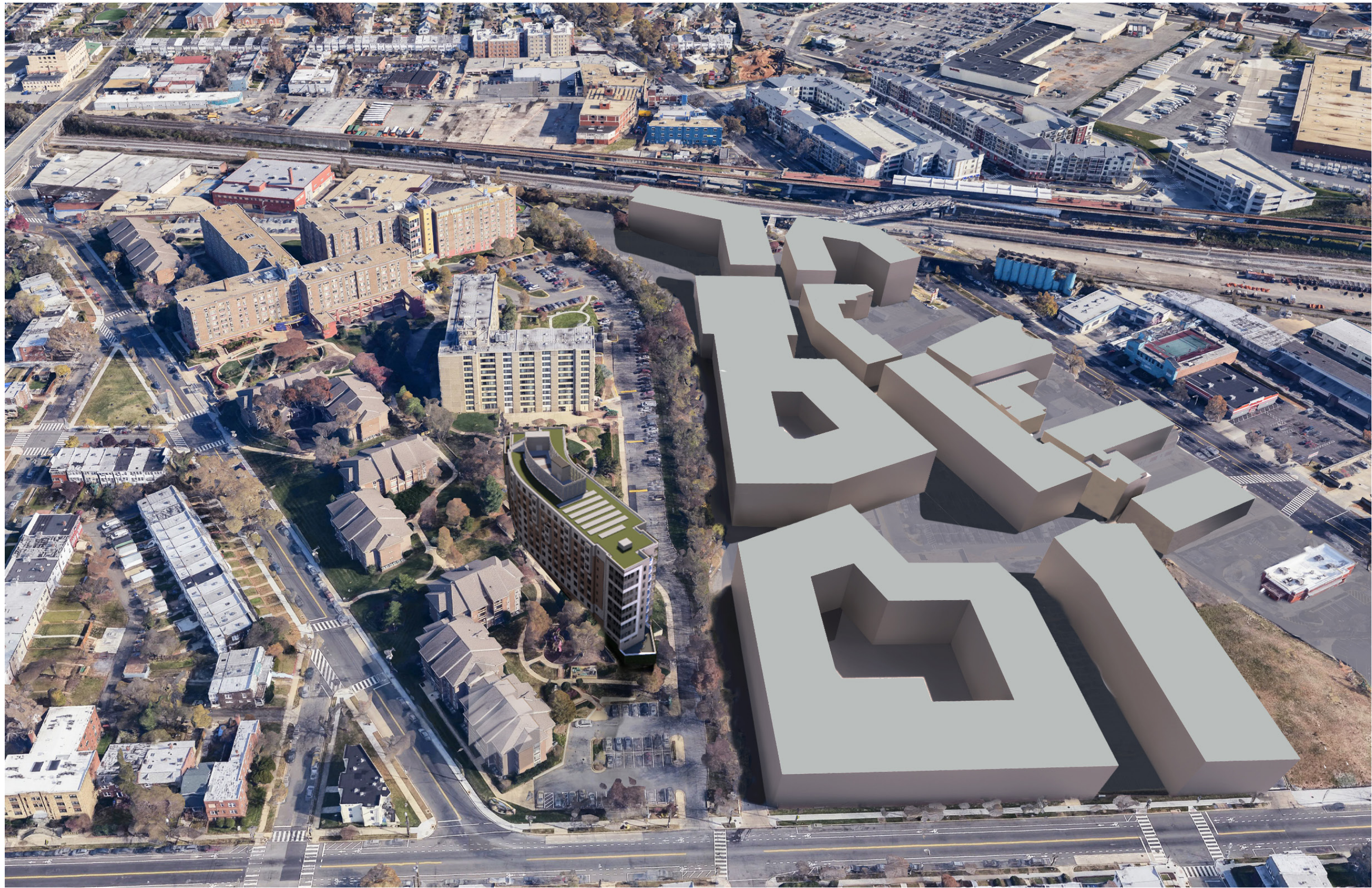
View From the West
